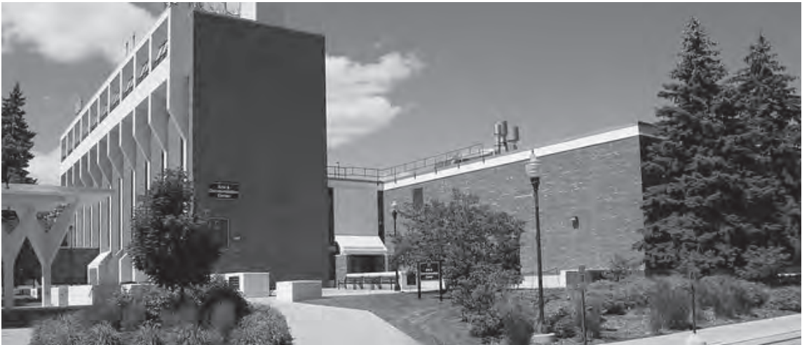
Courtesy of UWO The Arts and Coummunications building, which is near where the gas leak happened on Jefferson Street.
